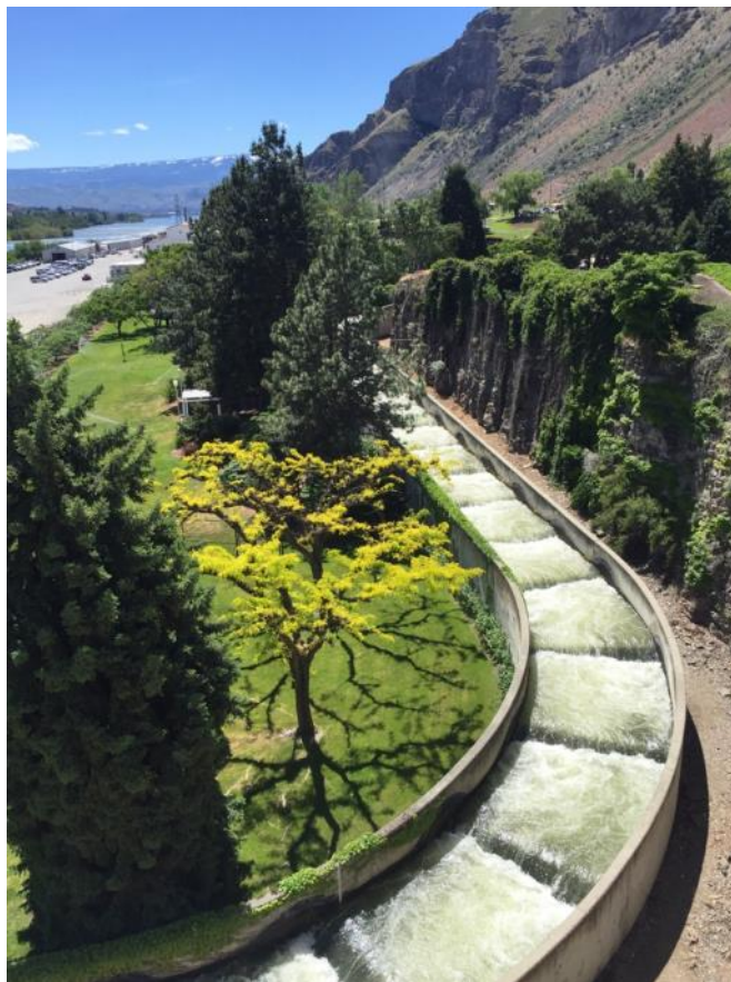
Rocky Beach Dam's gorgeous fish ladder, located in Chelan County, WA.
